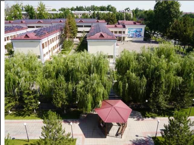
1. Each building of the university is equipped with solar panels (UzSWLU)
