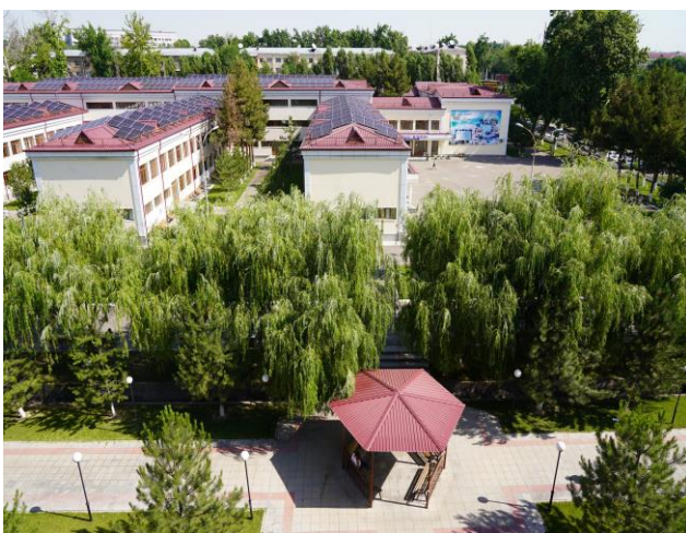
Each building of the university is equipped with solar panels (UzWSLU)
