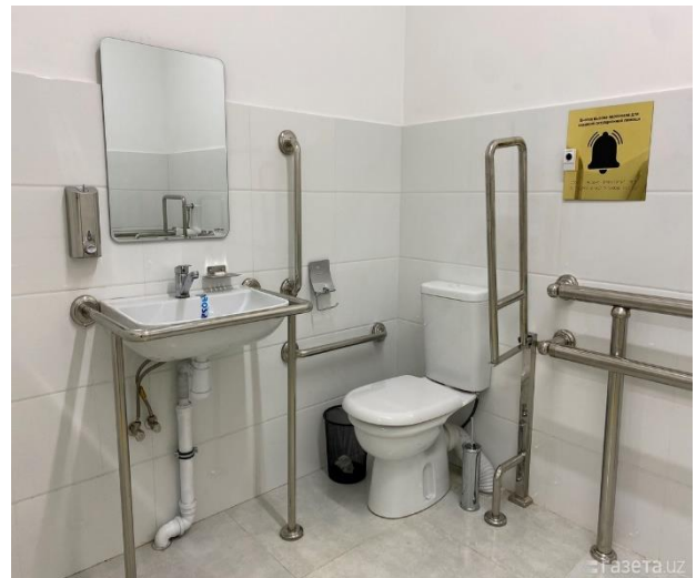
Toilets for students with disabilities
