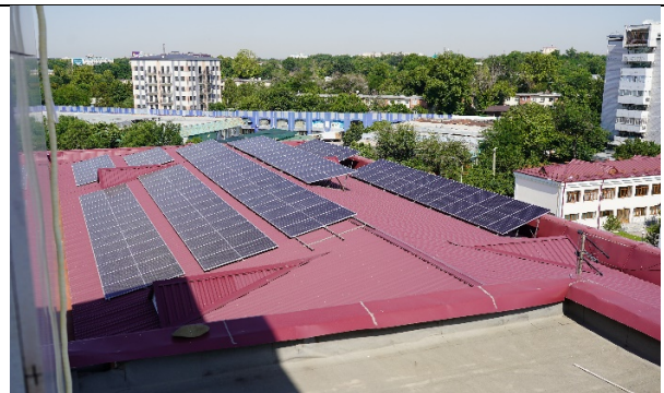
Rooftop solar PV installation
