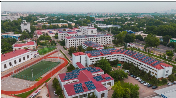
Rooftop solar PV arrays at UzSWLU
